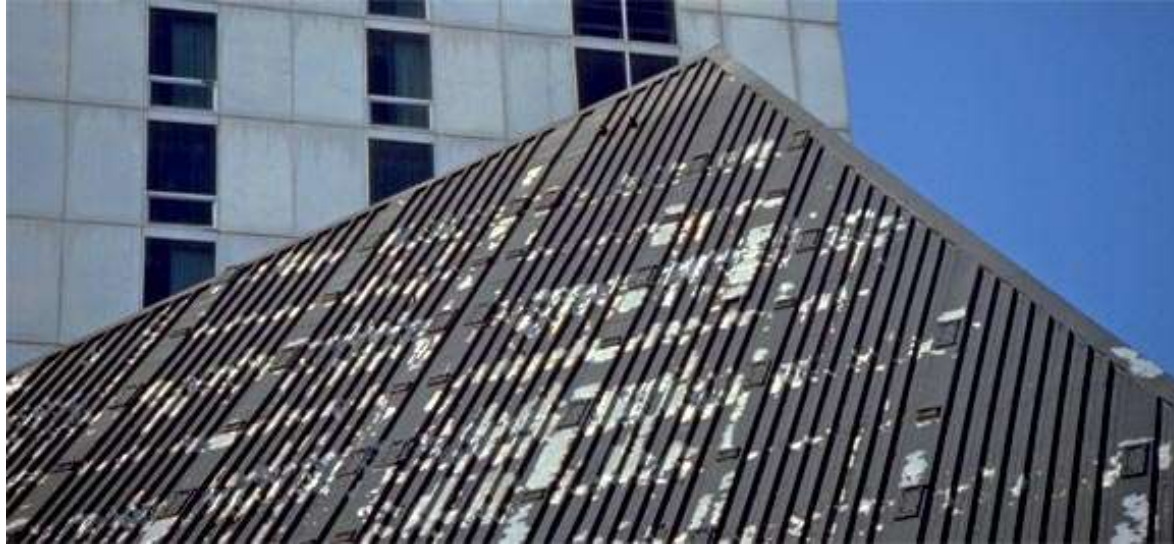
Peeling painted aluminum roof, 25 years
