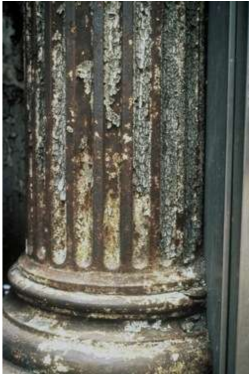
Peeling painted carbon steel
